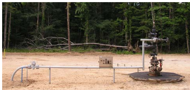
CO 2 -EOR production wellhead at a SECARB test site. (Courtesy: BEG, UT Austin)
